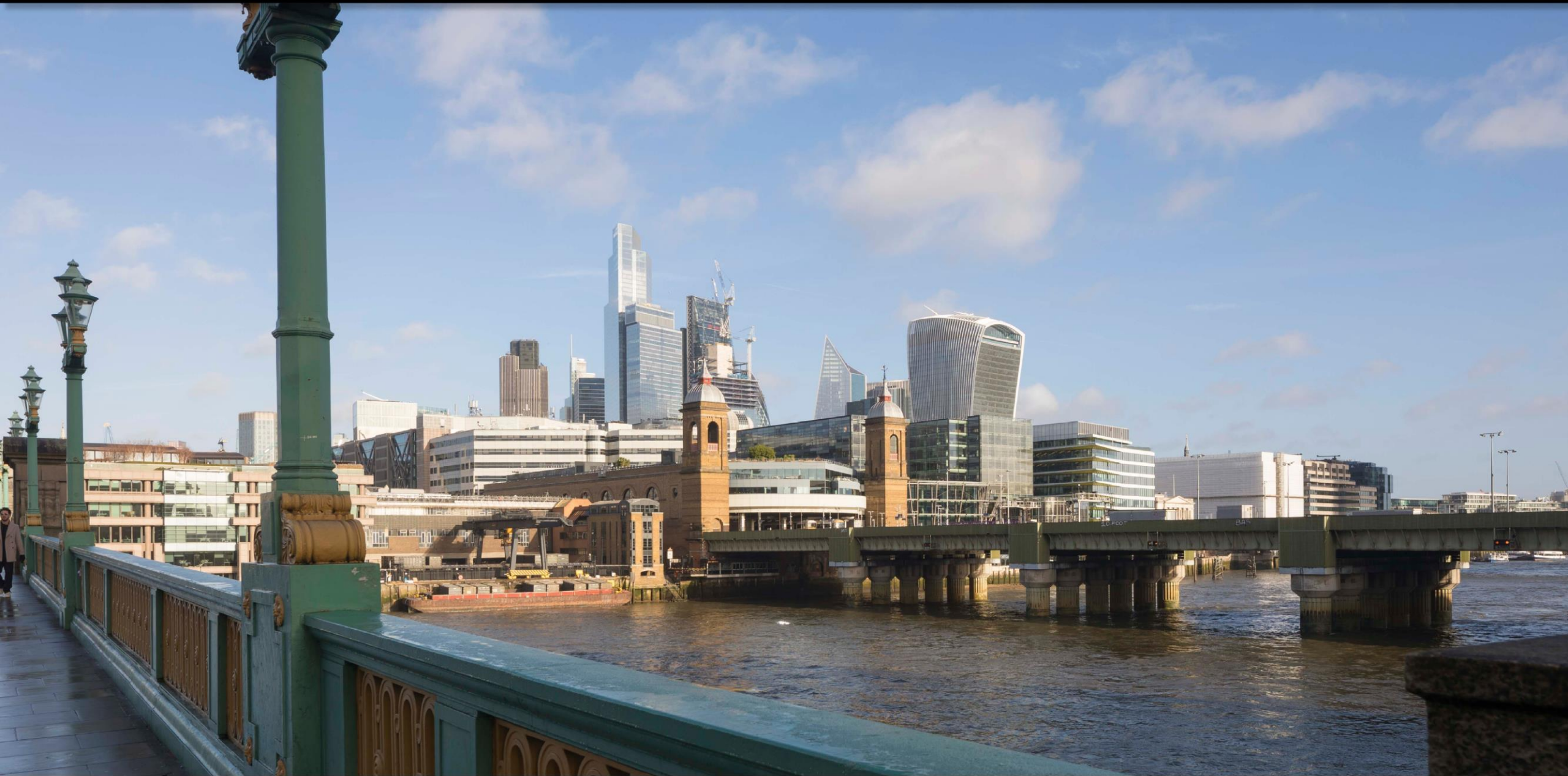
Southern end of Southbank Bridge
