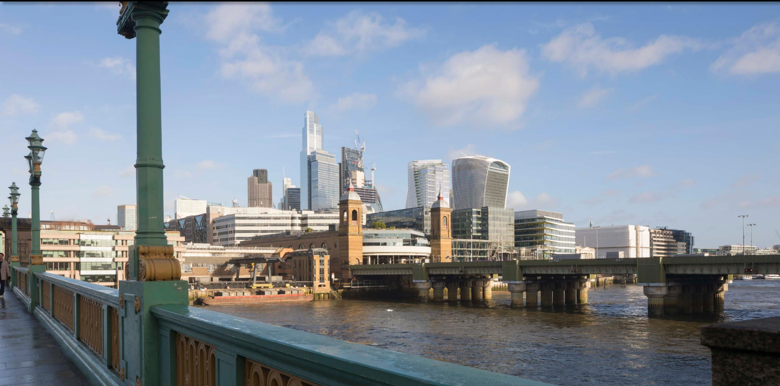
Southern end of Southbank Bridge
